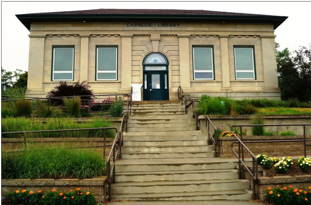
Ponca Carnegie Library
